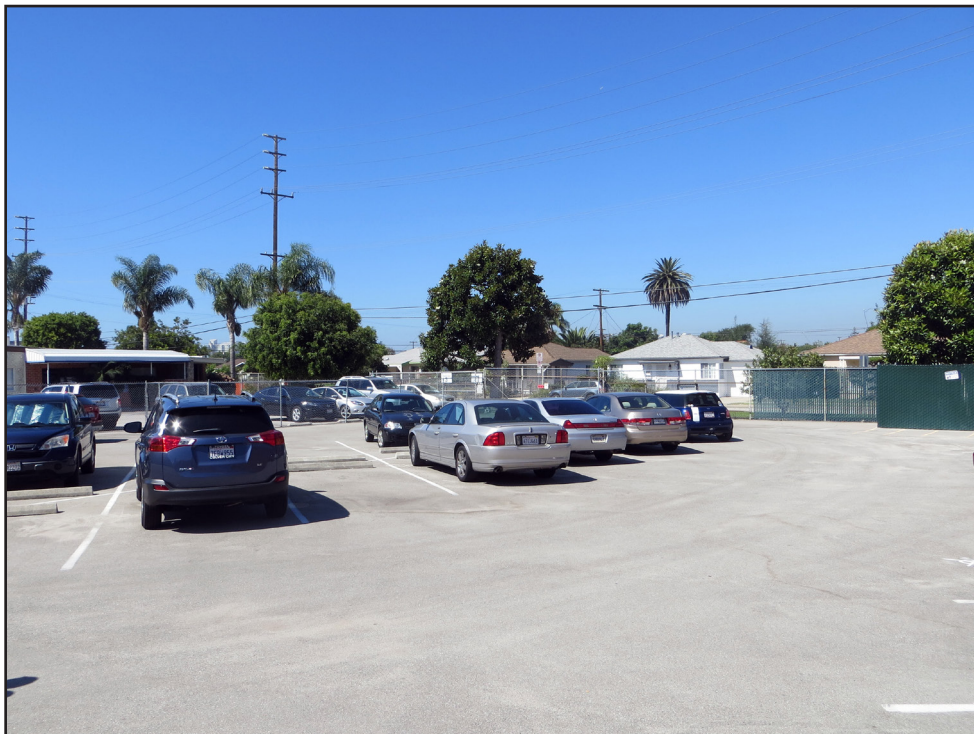
Photo 2. View looking west across north parking lot toward Panama Street.
