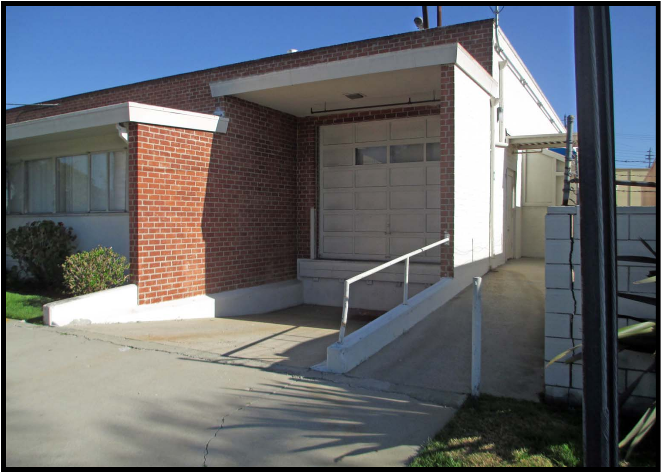
Loading Dock on Southwestern Corner of Existing Building (ESE)
