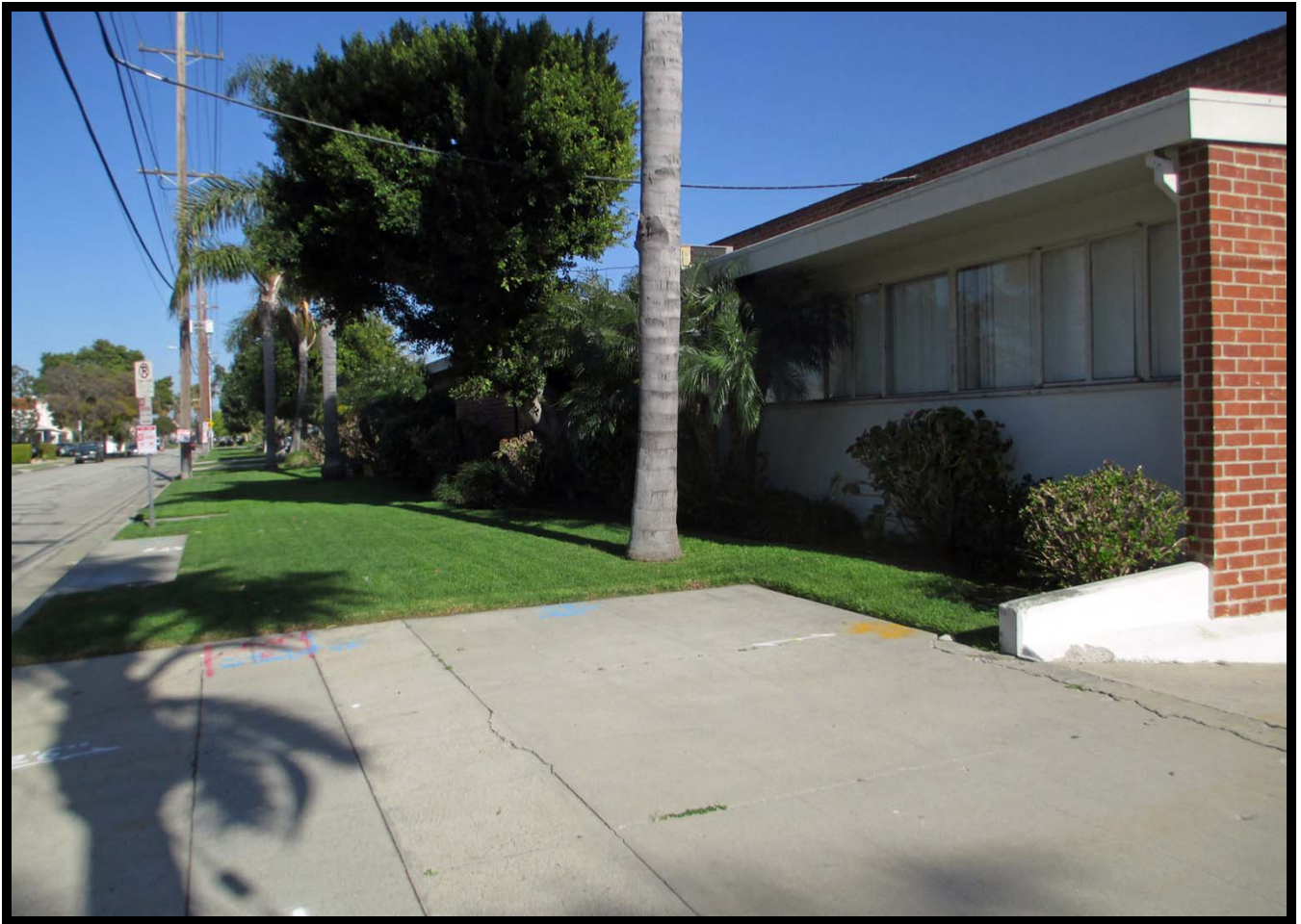
Overview of Western Elevation of Existing Building (NE)
