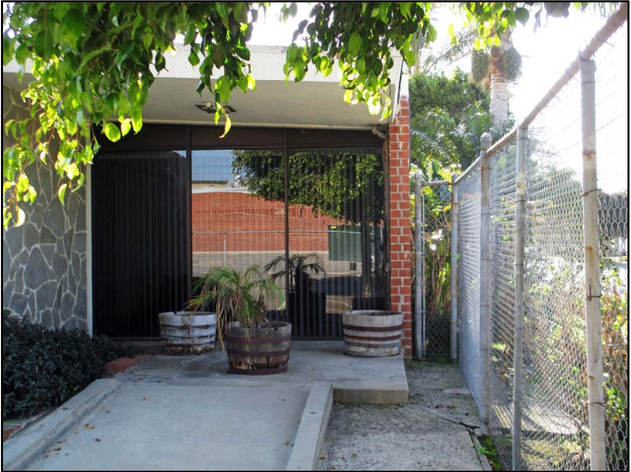
Figure 8. Main Entry to the Building at 12870 Panama Street (South).
