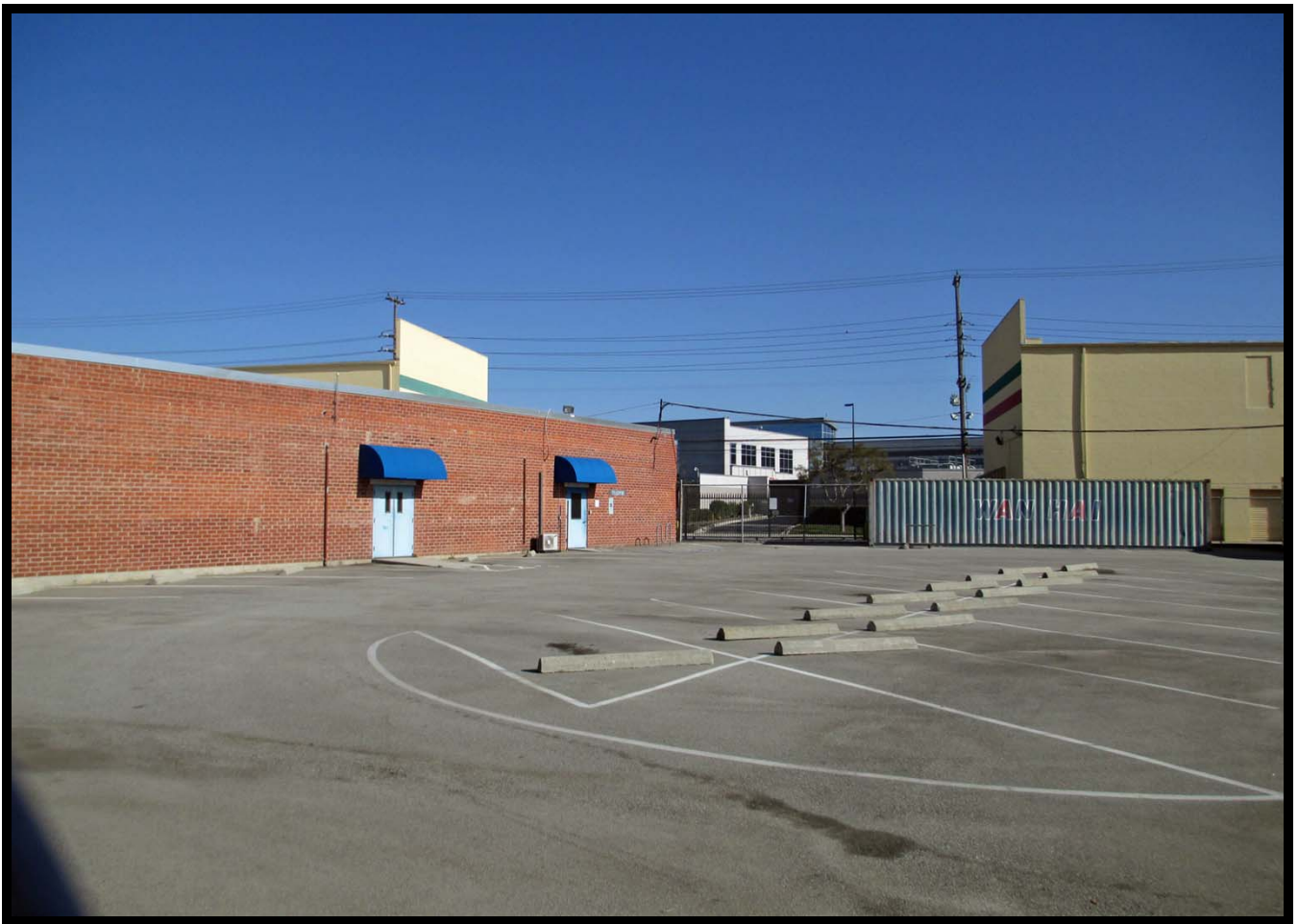
Employee Parking Lot Northeast of 12870 Panama Street and Southwest Elevation of Adjacent Property (NE)
