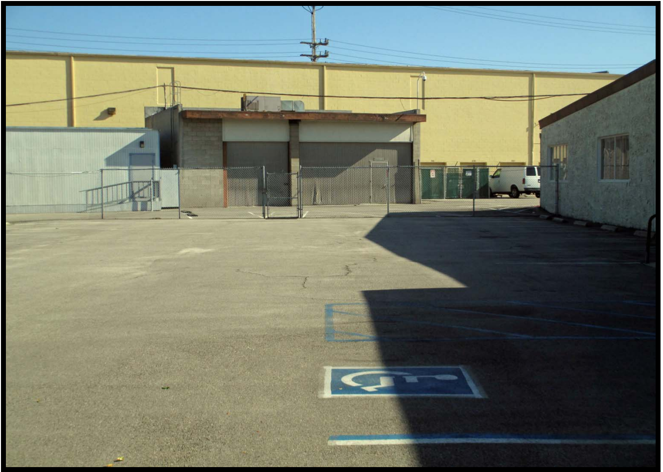
Ancillary Building behind 12870 Panama Street (SE)
