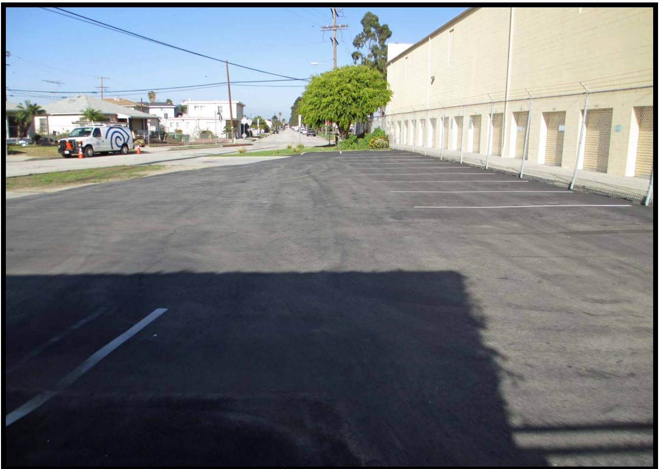
Parking Northeast of 12820 Panama Street (NE)
