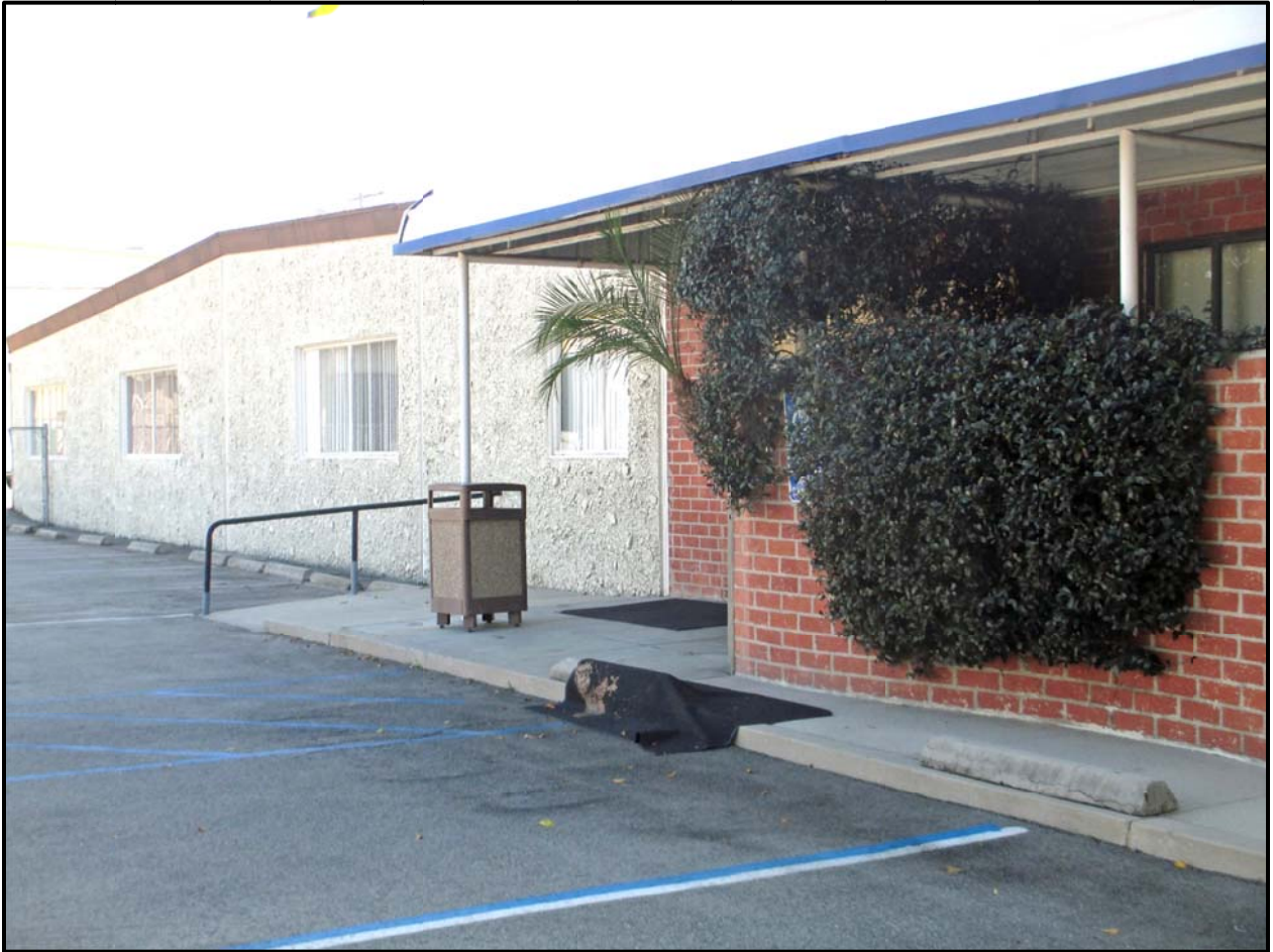
Figure 6. North Elevation of the Commercial/Industrial Building at 12870 Panama Street (ESE).
