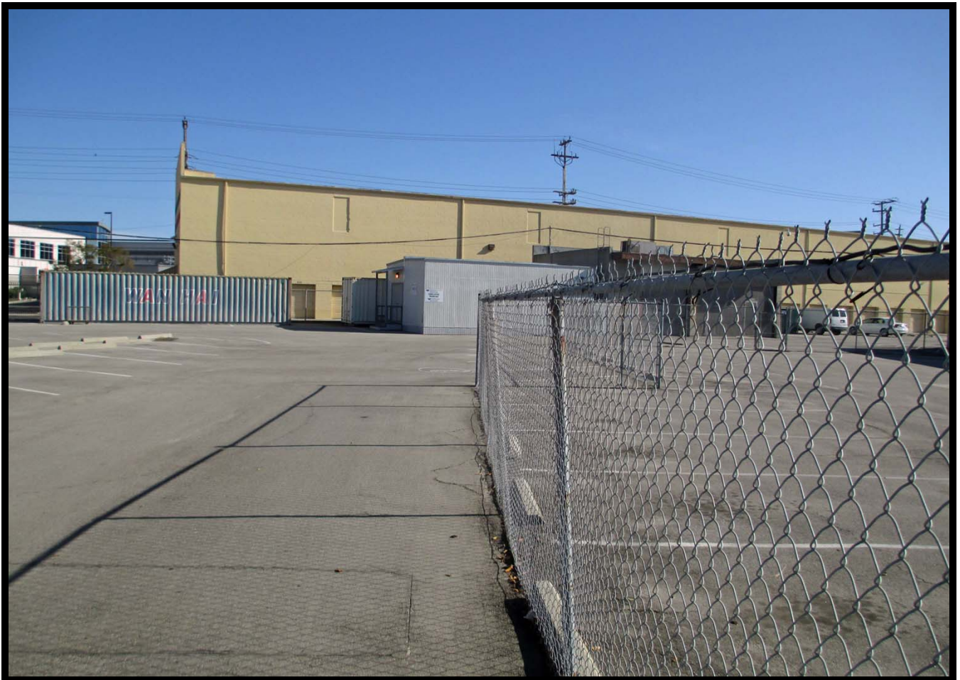
Employee Parking Lot Northeast of Building at 12870 Panama Street (SE)
