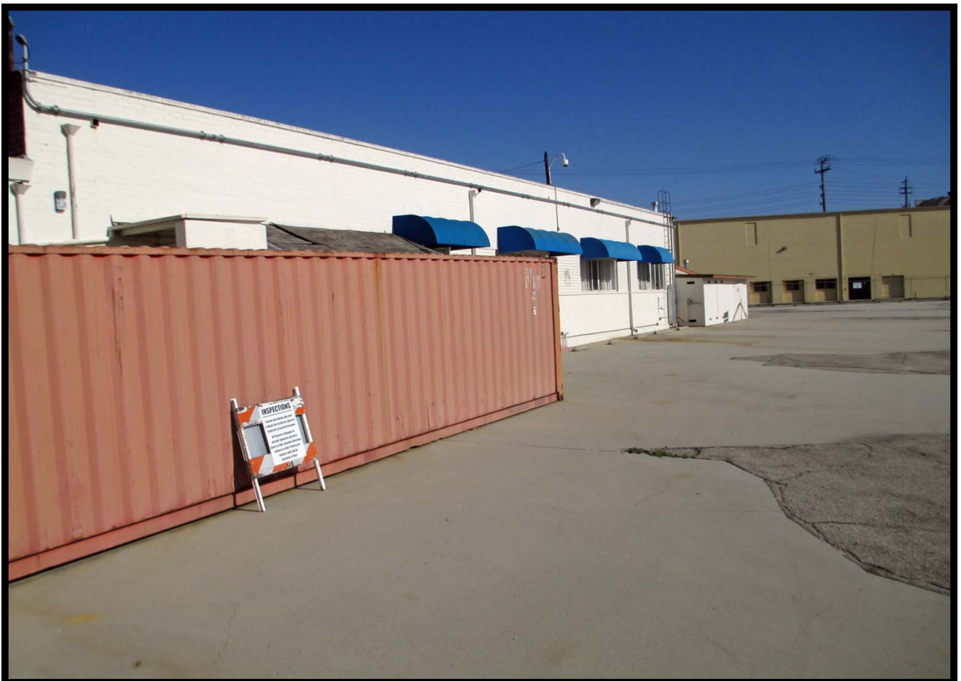
Southwestern Elevation of Existing Building (E) with Storage Container in Yard
