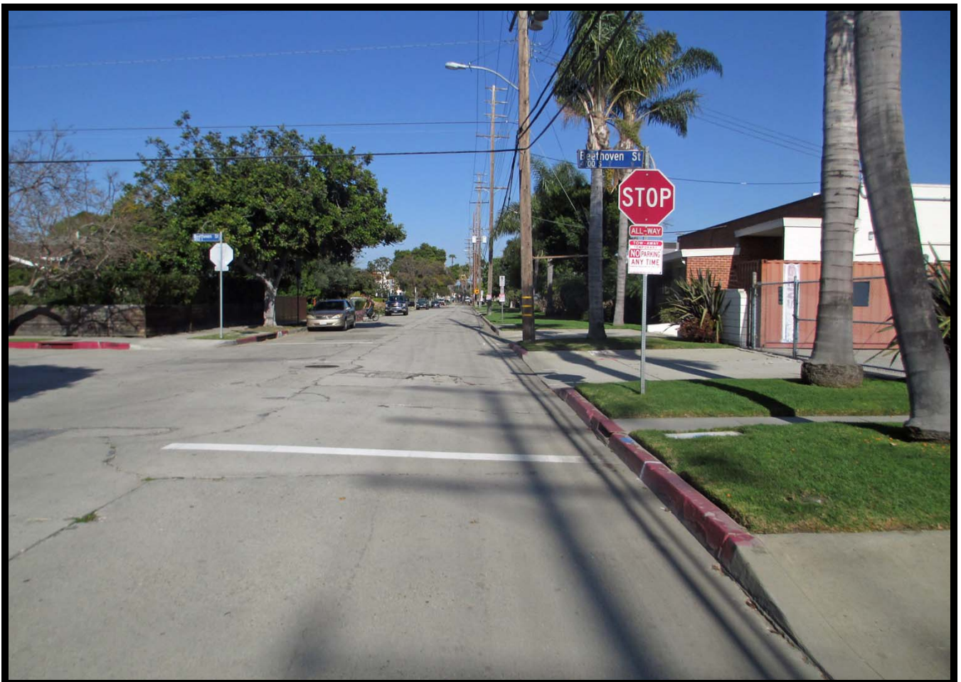
Overview of Panama Street from Beethoven Street (NE)
