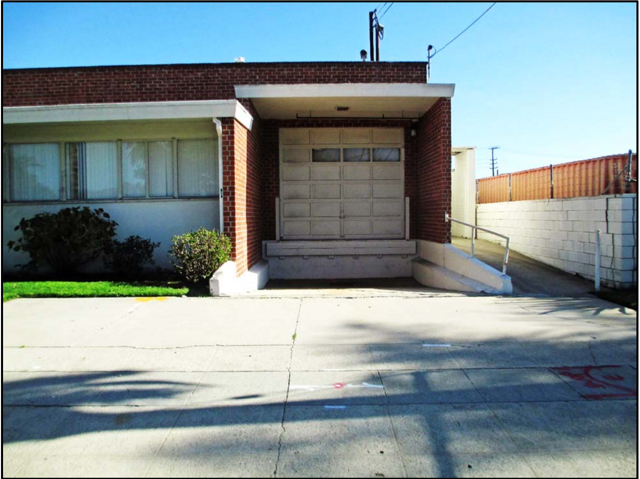
Figure 7. Southwest Corner of Building with Loading Dock facing Panama Street.
