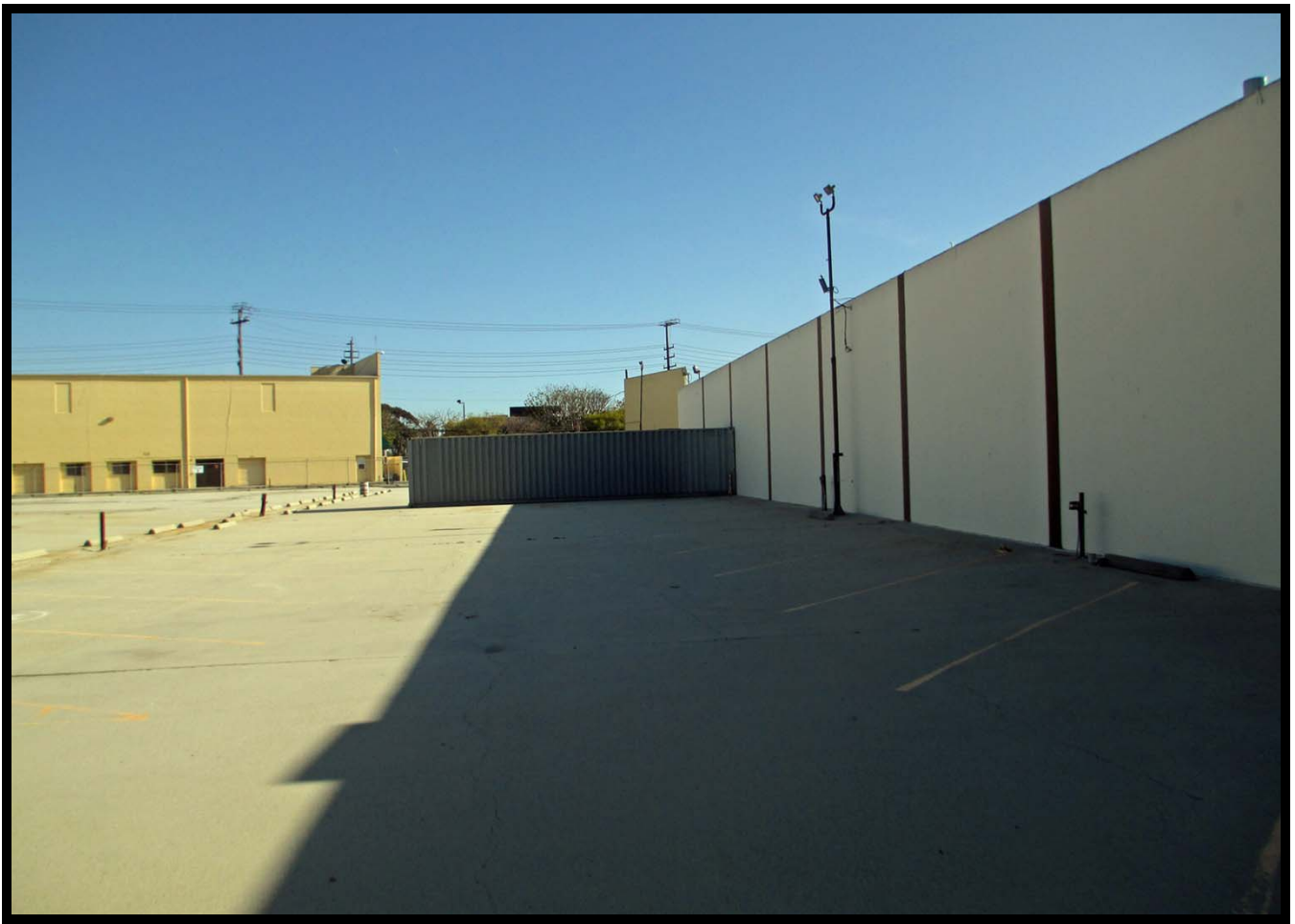
Southern Parking Surface, Opposite Beethoven Street (SE)
