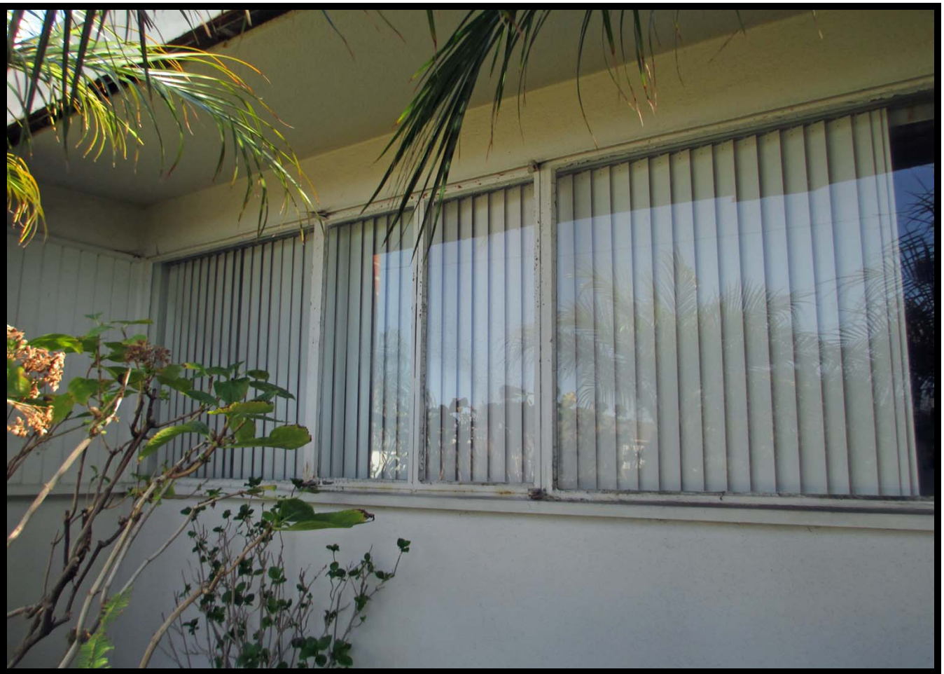
Detail of Casement and Fixed Windows on Western Elevation (ENE)
