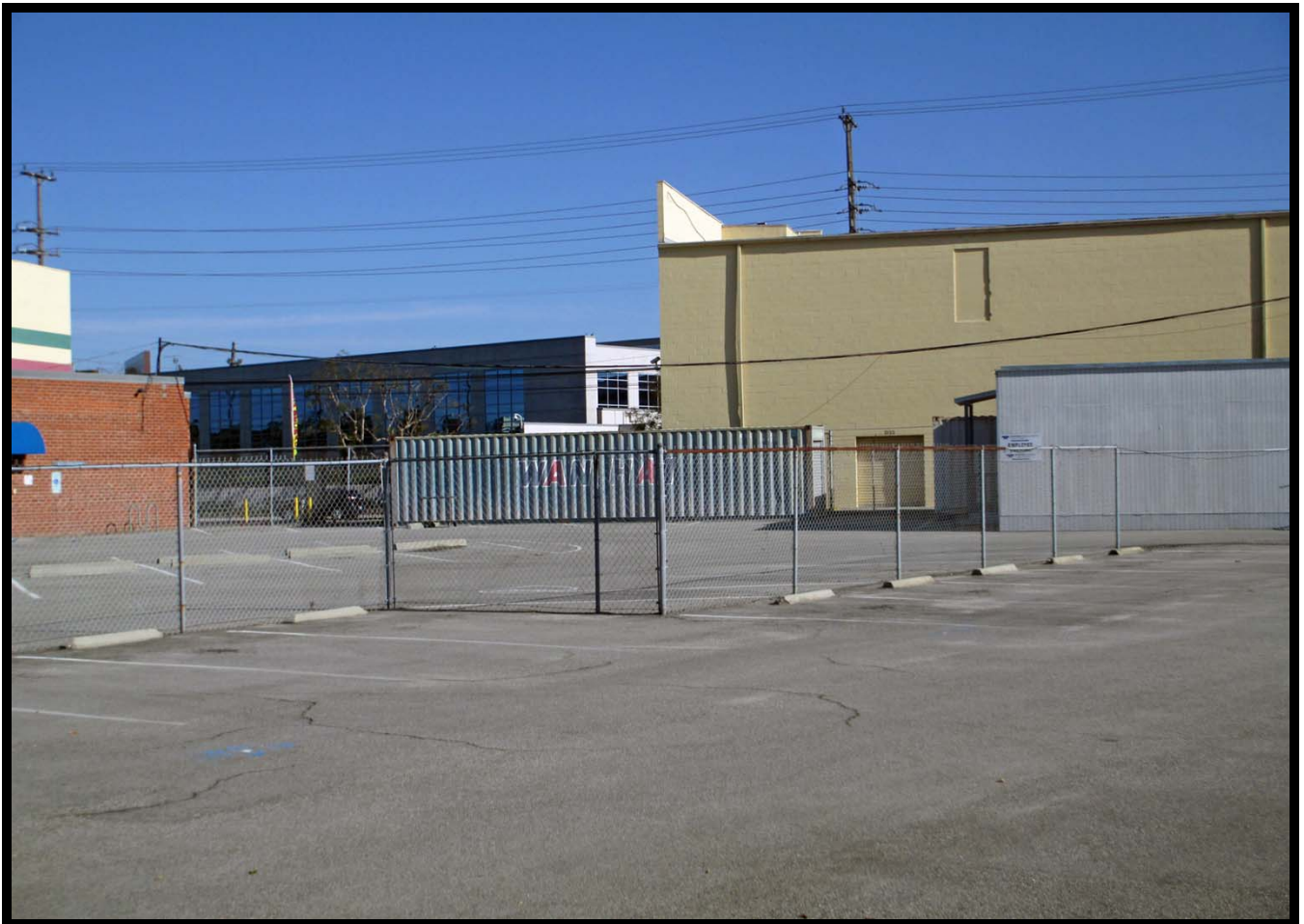
Storage Areas in Parking Lot Northeast of 12870 Panama Street (E) G-90
