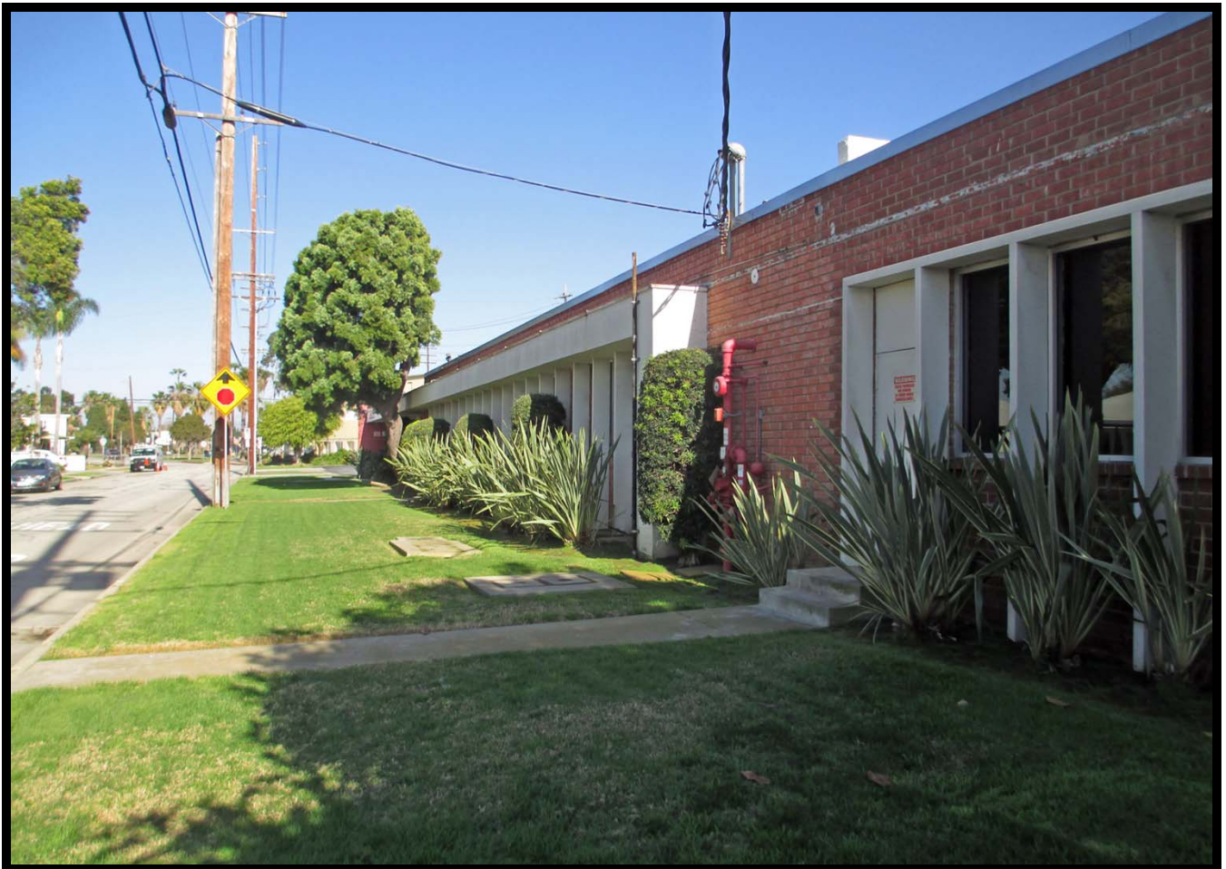
Teledyne Building at 12820 Panama Street (NNE)
