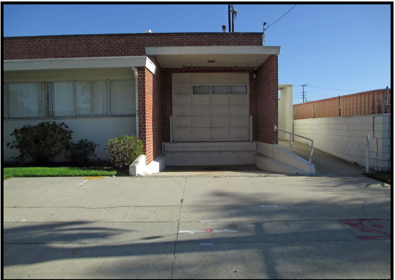
Overview of Loading Dock on Panama Street (SE)
