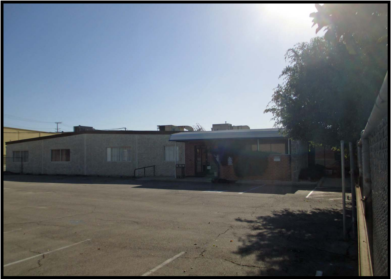
Northern Elevation of Building at 12870 Panama Street (SW)
